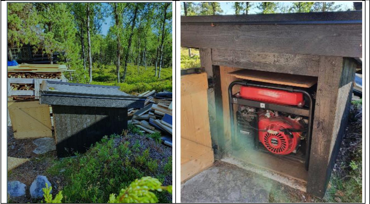
Overbygg for aggregat.
