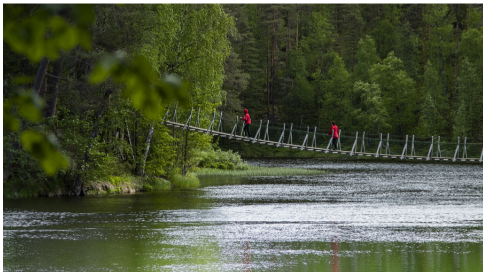
Suspension bridge at Harrisuvanto on Karhunkierros hiking trail. PHOTO: Metsähallitus
